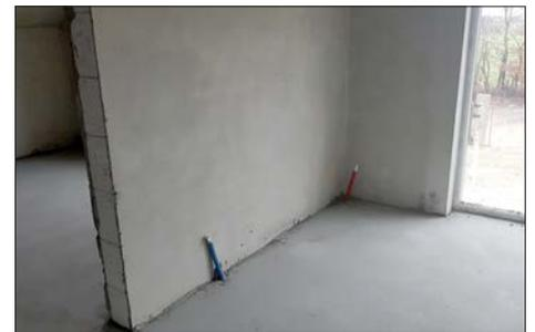
*Pipes for the heating system for the second floor. Even the basement has been cast.*
